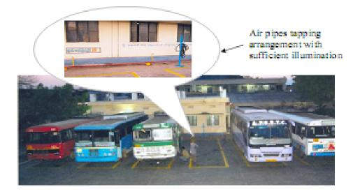
The materials required for air tapping at the exclusive inflation bay are GI Pipes of suitable length, Pipe connectors, hose pipes and Quick-on couplers. The Quick-on couplers are stock item at most of J-wards and may be procured to the required quantities, if not. The hand pressure gauges or mobile wall pressure gauges can be used for checking the tyre pressure at the bays.
